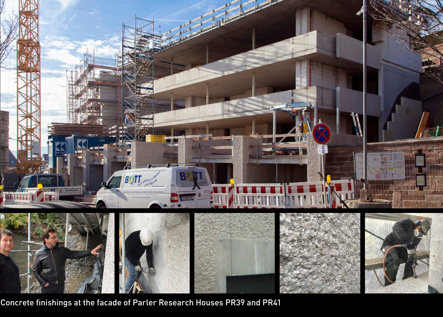
Concrete finishings at the facade of Parler Research Houses PR39 and PR41
