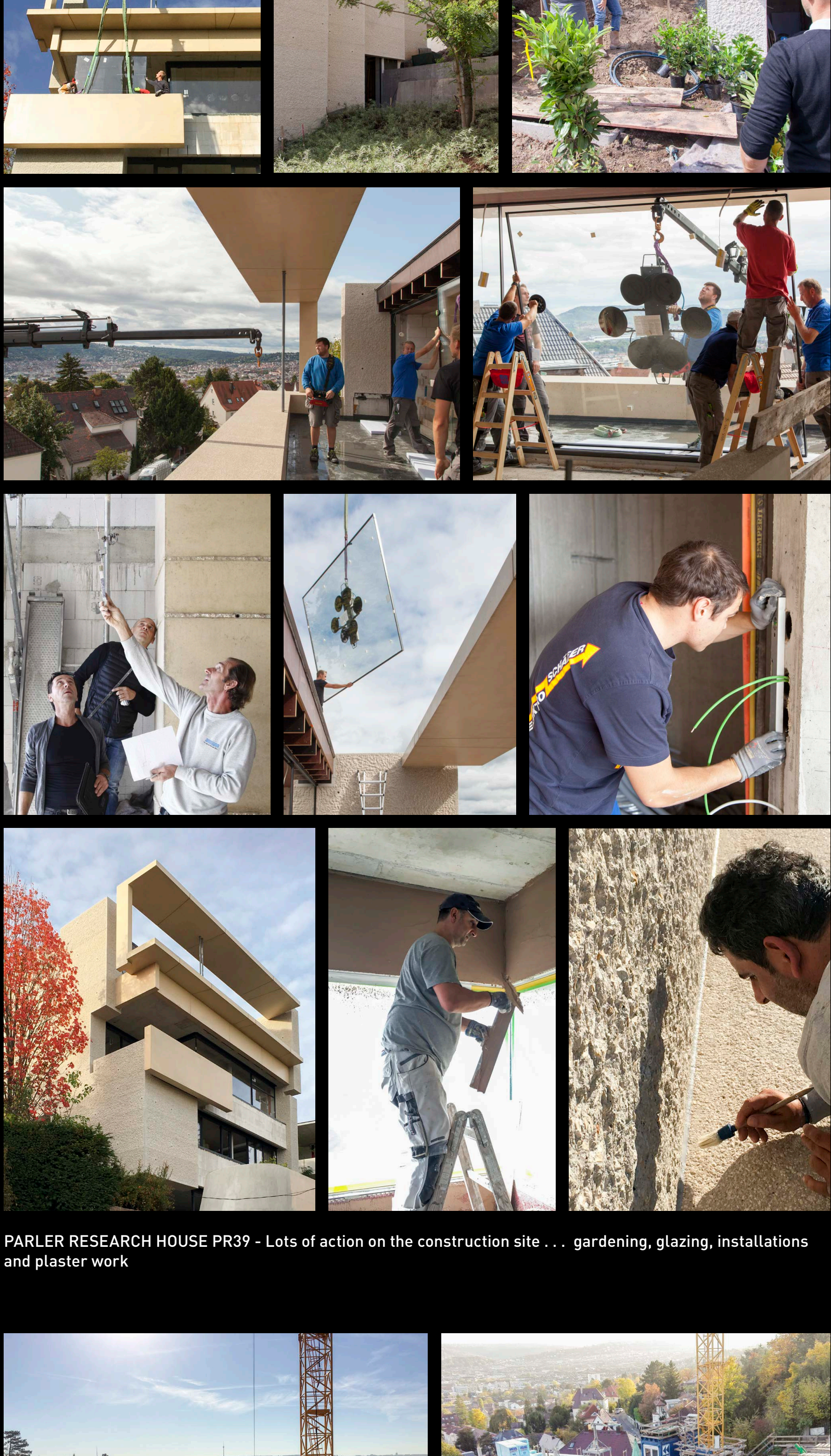
PARLER RESEARCH HOUSE PR39 - Lots of action on the construction site . . . gardening, glazing, installations and plaster work
